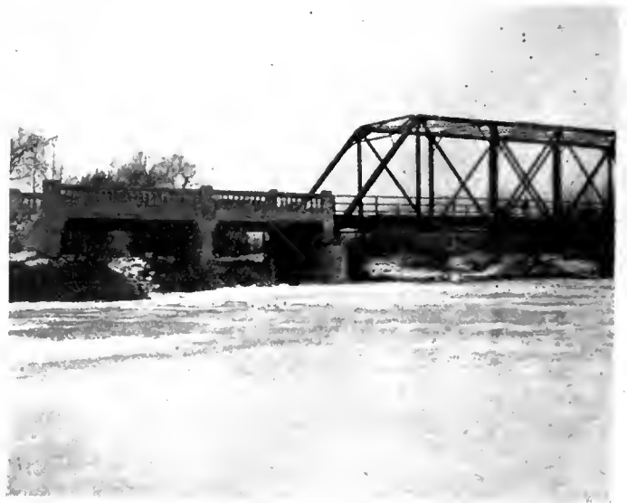
Valley River bridge—110 ft. steel truss with two 25 ft. concrete approach spans
